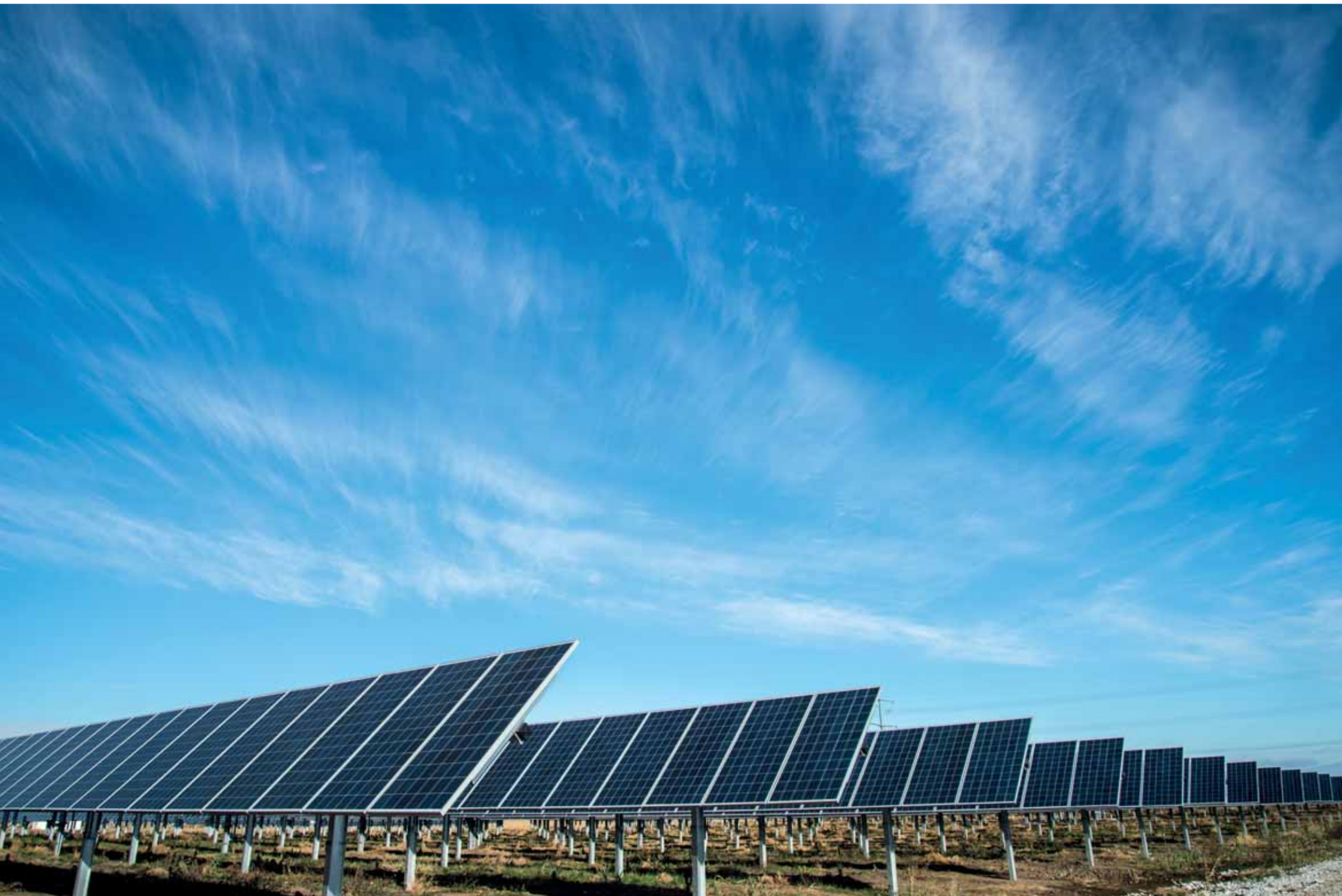
Tracker panels can follow the sun through the day, maximising generation
